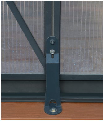
Internal ground anchoring system
